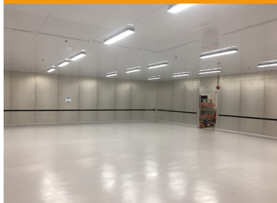
Epoxy flooring in cooler
