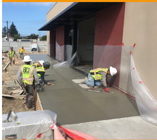
Pathway/ sidewalk at Training Classroom
